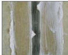
Brush the paste into the surface. Then apply OTTOSEAL® StainEx again.
