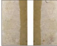
Mechanically remove the sealant completely from the joint.
