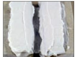
Use a putty knife spreading the paste evenly, creating a layer of min 5 mm.
